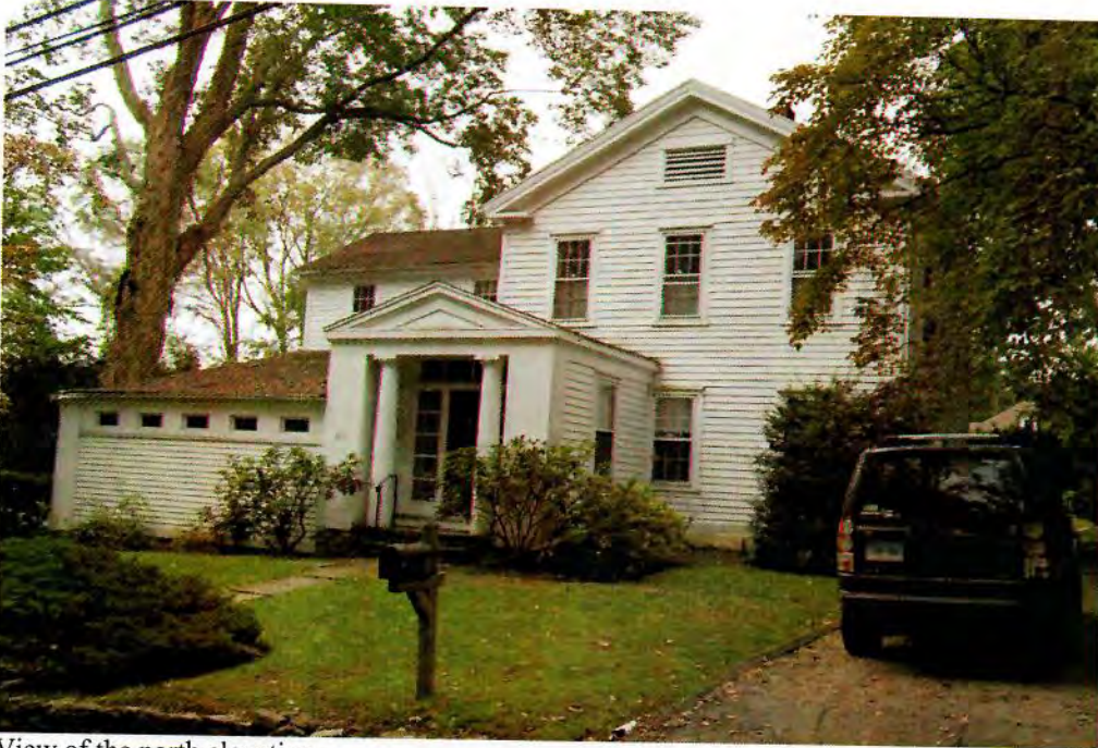
View of the north elevation.
