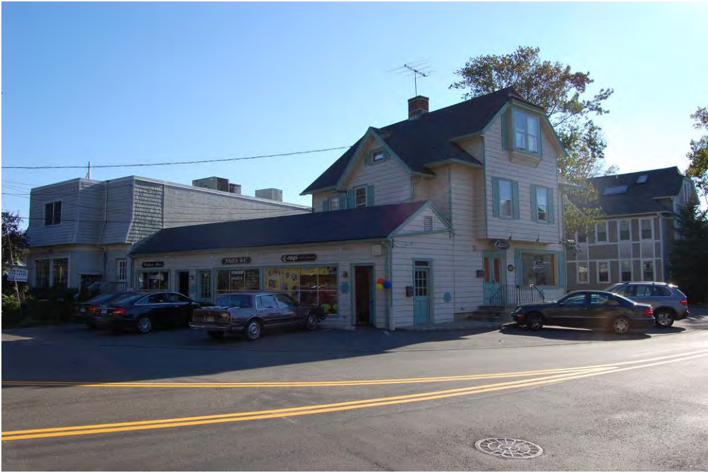
View of the north and east elevations.
