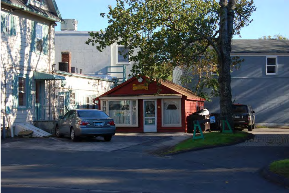
View of the converted garage.
