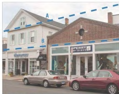
Figure 36E Roof Parapet and Cornice Lines
