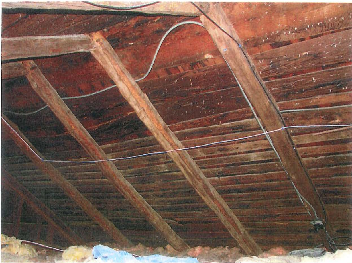
Photo 4. Attic and interior roof structure.
