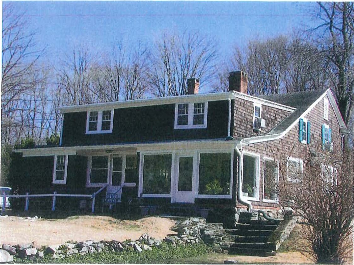
Photo 2. Northwest and west elevations, view south.
