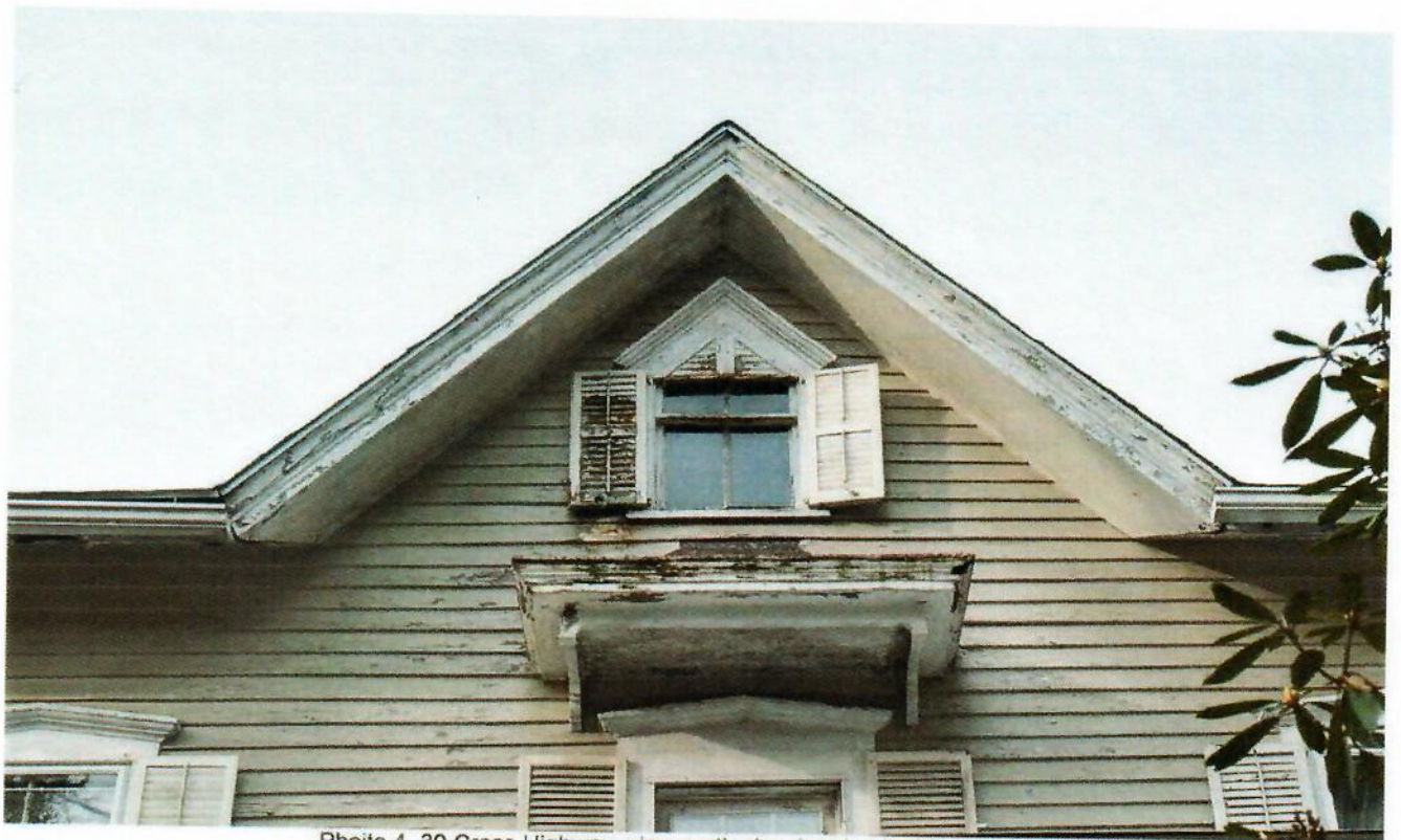
Photo 4. 39 Cross Highway, view north showing detail of facade gable.
