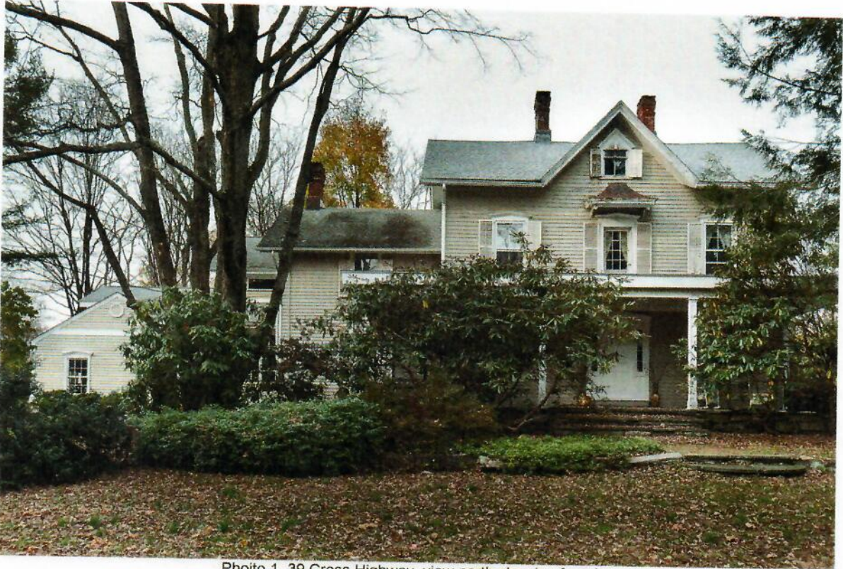
Photo 1. 39 Cross Highway, view north showing facade.
