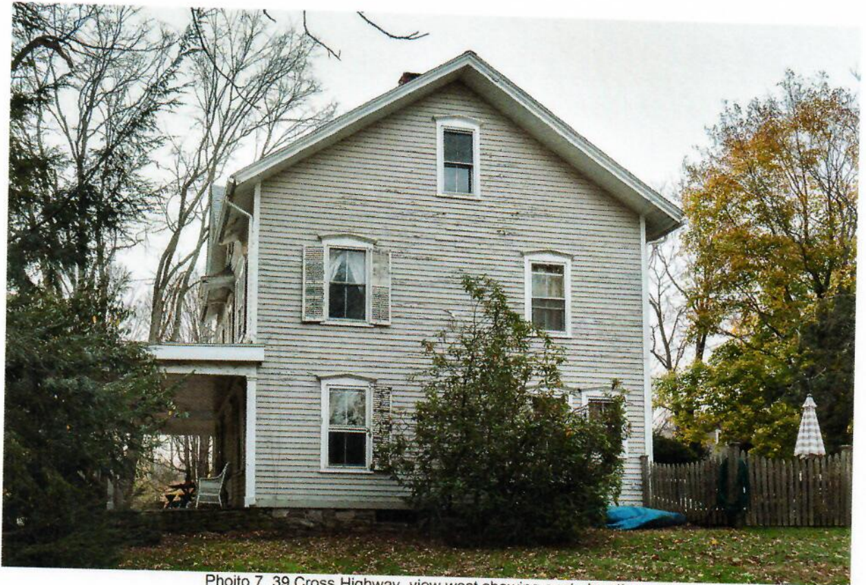
Photo 7. 39 Cross Highway, view west showing east elevation.
