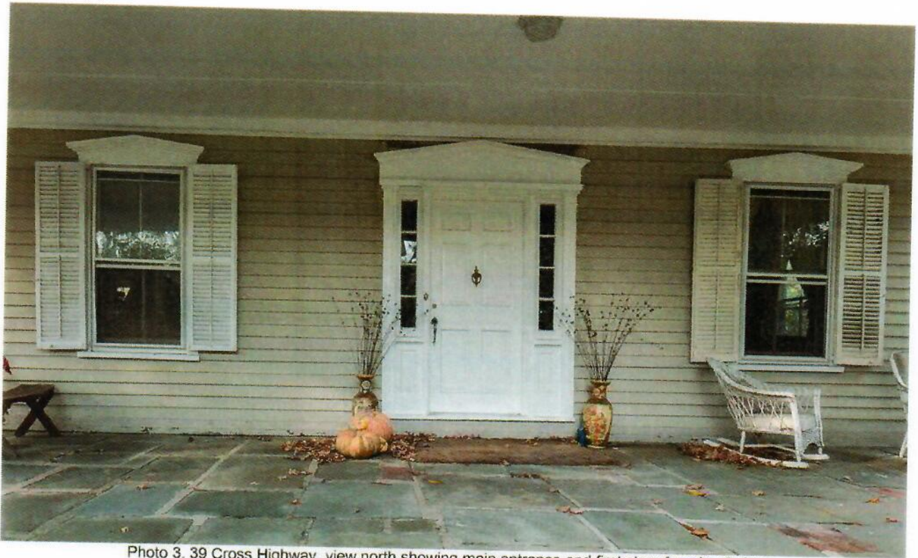
Photo 3. 39 Cross Highway, view north showing main entrance and first story facade windows.
