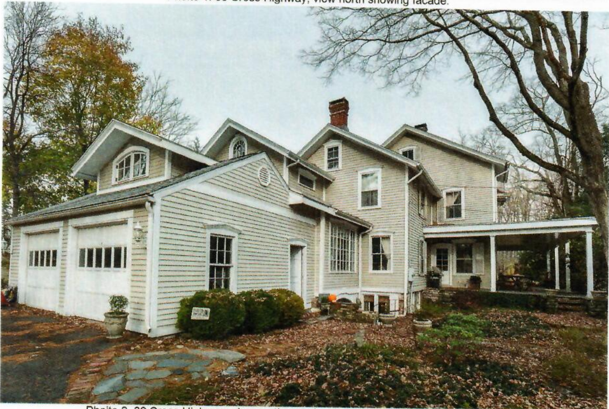
Photo 2. 39 Cross Highway, view northeast showing west elevation and part of facade.
