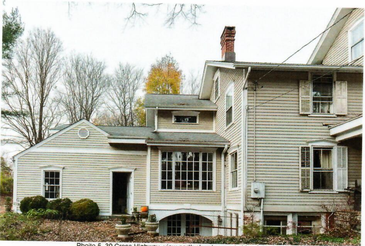
Photo 5. 39 Cross Highway, view north showing west side of facade.
