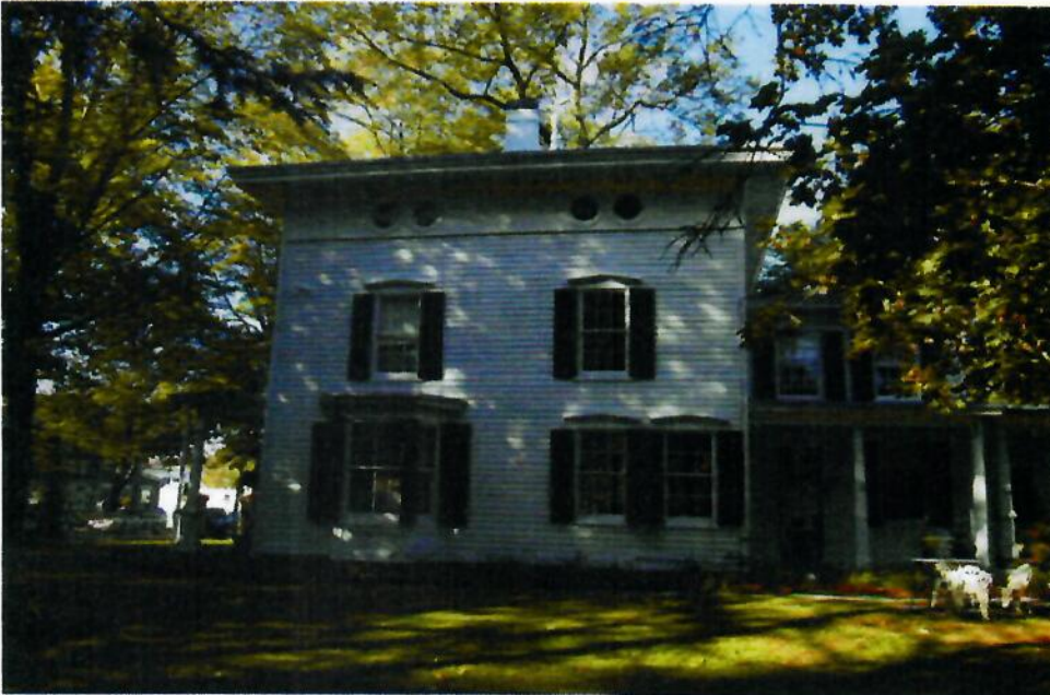
View of the east elevation.
