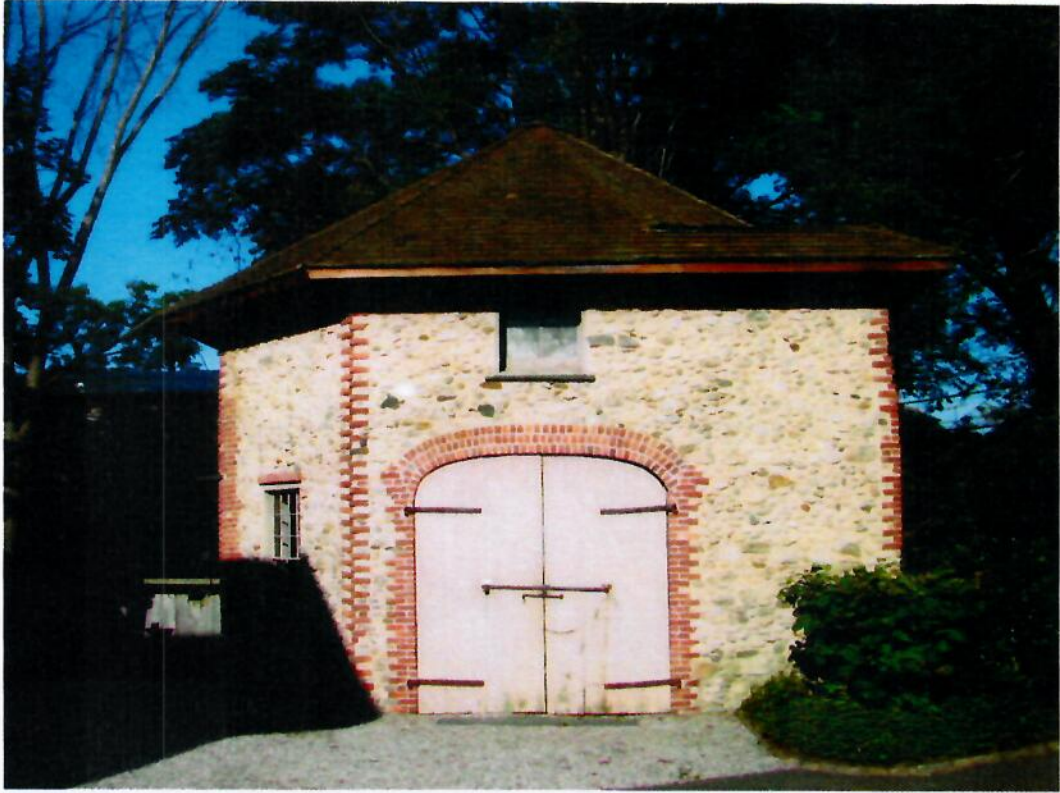
Figure 5: Cobblestone Barn – entrance/east side (2012)
