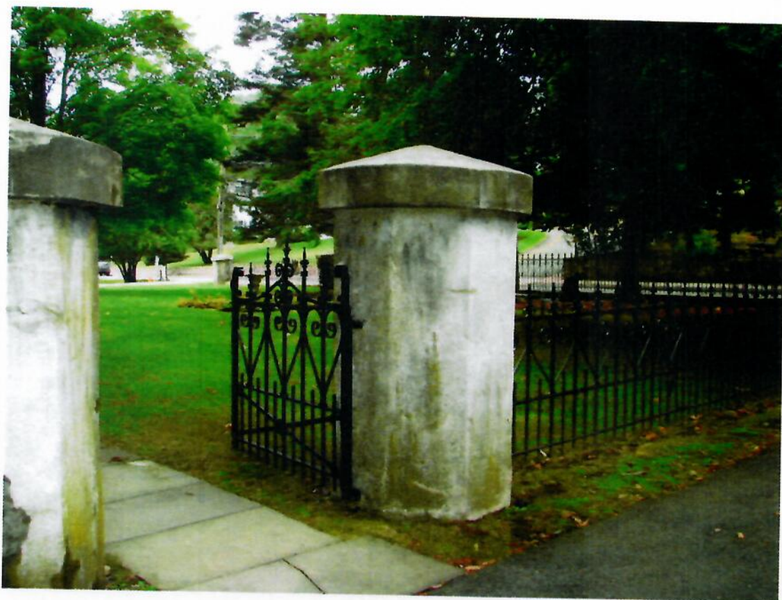
Figure 7: Polygonal Stucco Post with Wrought Iron Fence (2012)
