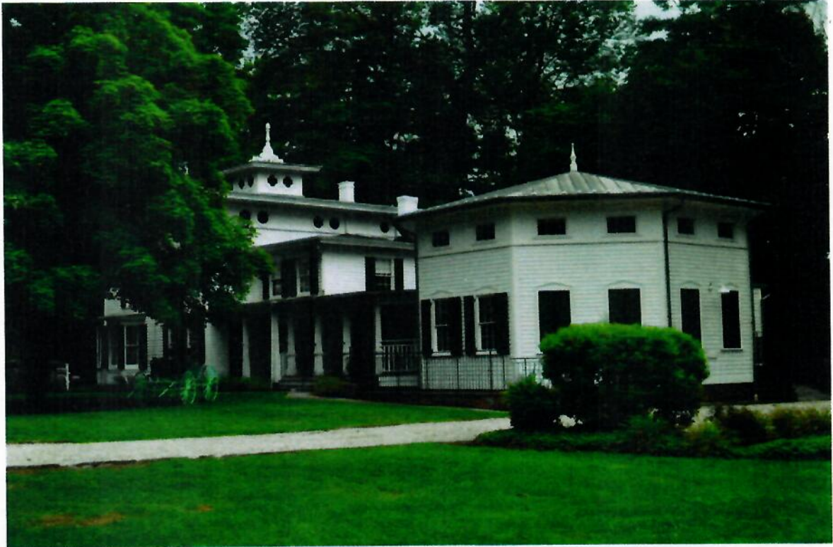
Figure 3: North and East Sides - 2012
