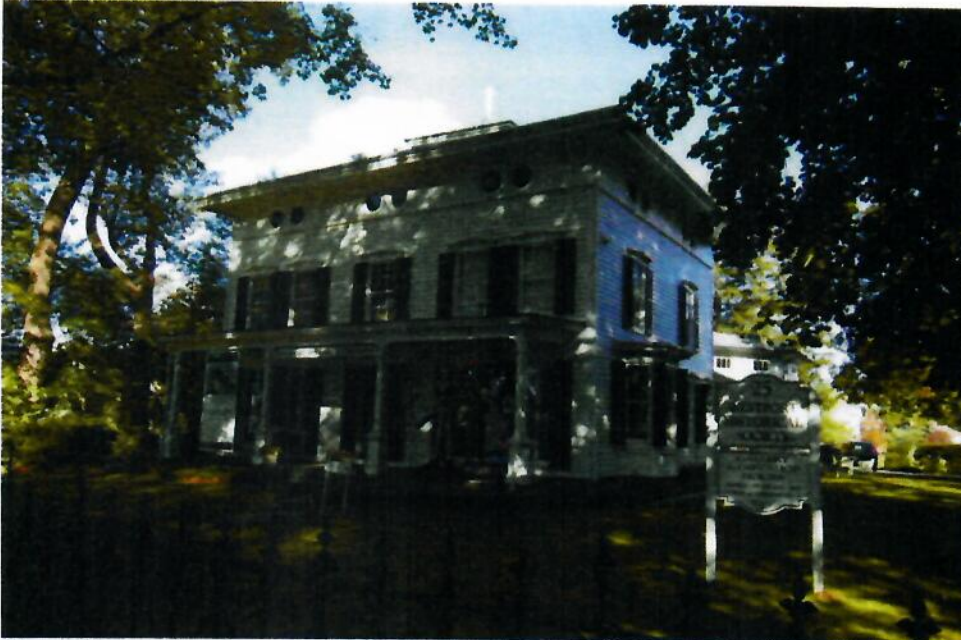
View of the south and east elevations.
