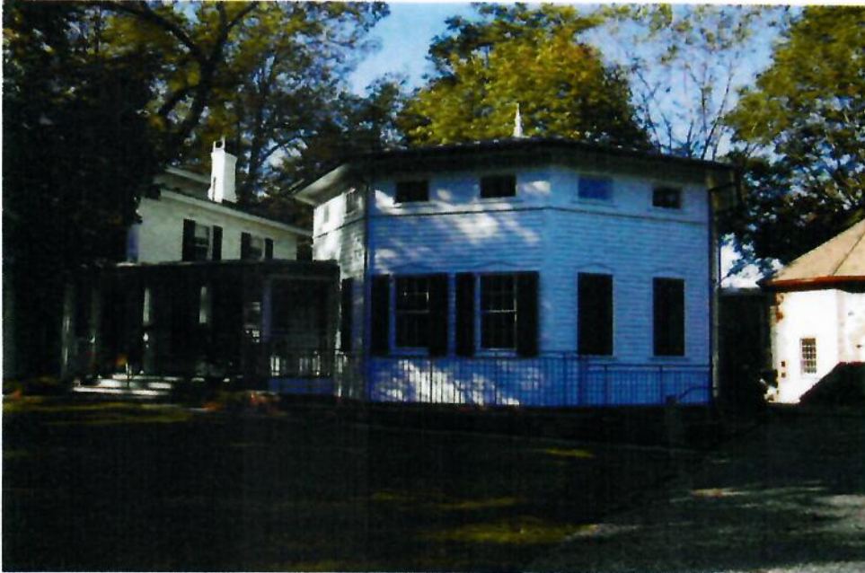
View of the east elevation.
