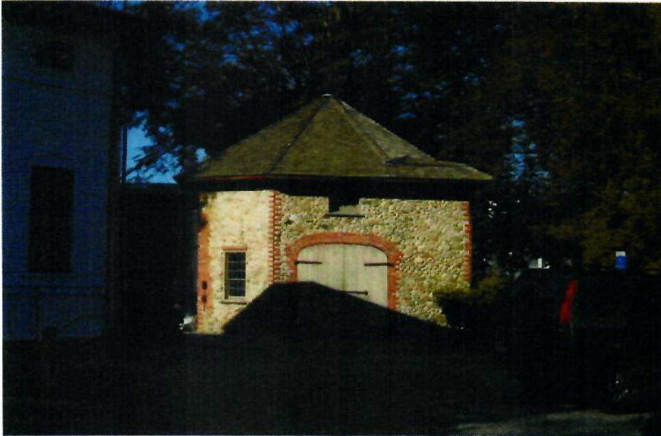
View of the east elevation of the carriage house.
