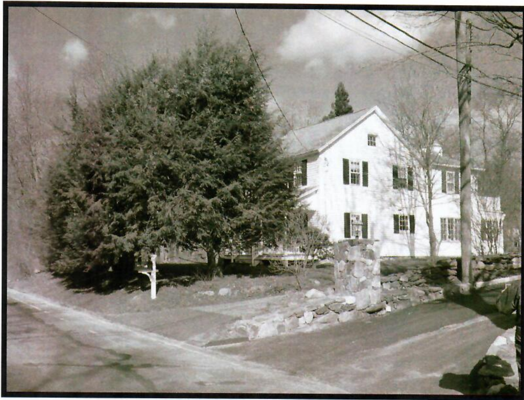
Figure 2. Main House—View to Northeast
