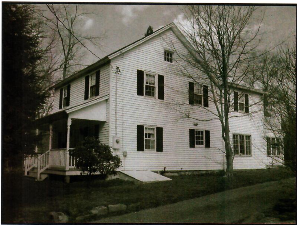
Figure 4. Main House—View to Northeast
