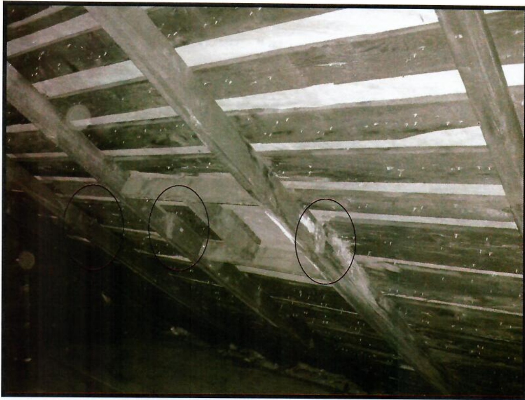
Figure 20. Roof Framing Detail with Original Rafter Ends
