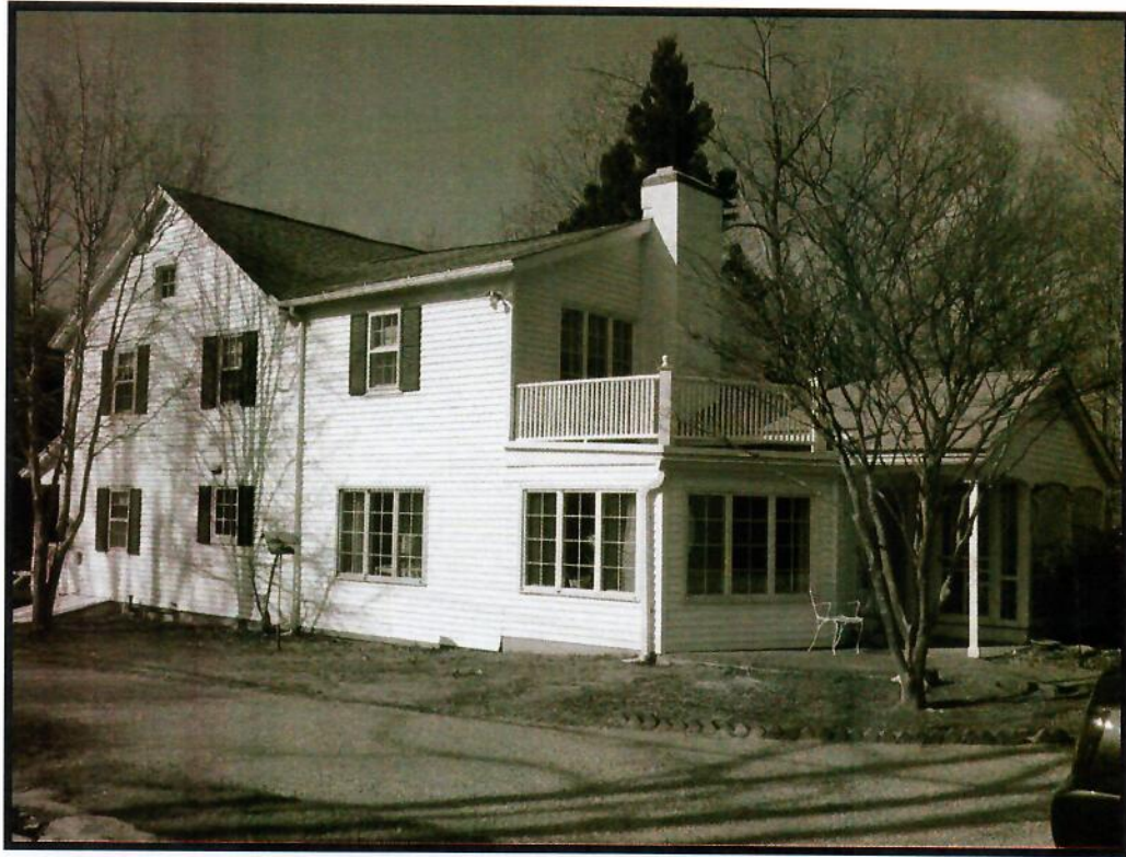
Figure 6. Main House—View to Northwest
