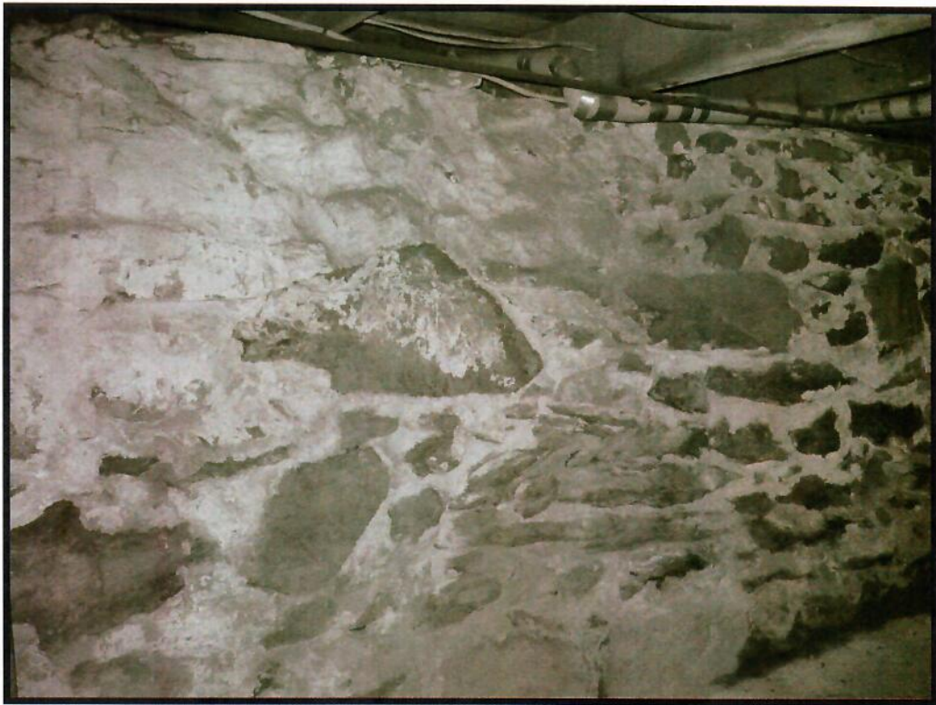
Figure 15. Foundation Wall Detail—View to Northwest
