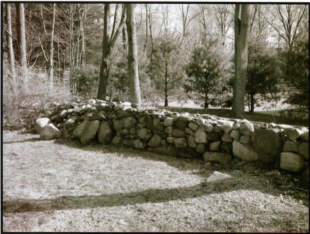
Figure 9. Stone Wall Detail—View to Southeast
