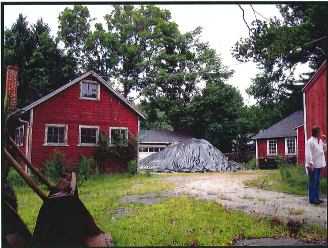
Figure 5. Auto Service Area—View to Northeast
