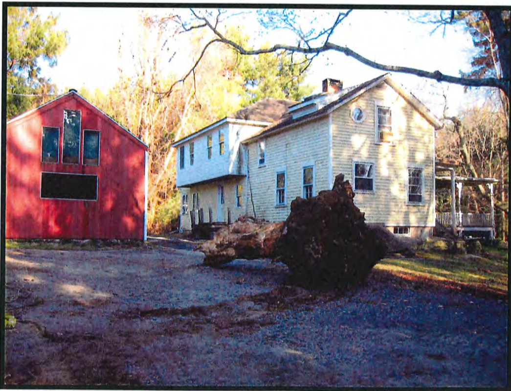
Figure 3. Main House & Converted Barn—View to Southeast
