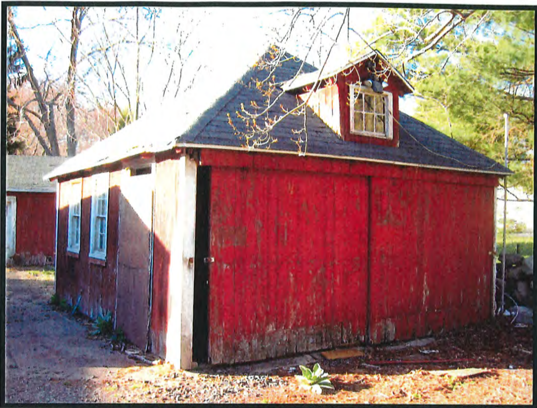
Figure 8. Garage Building—View to North [E]
