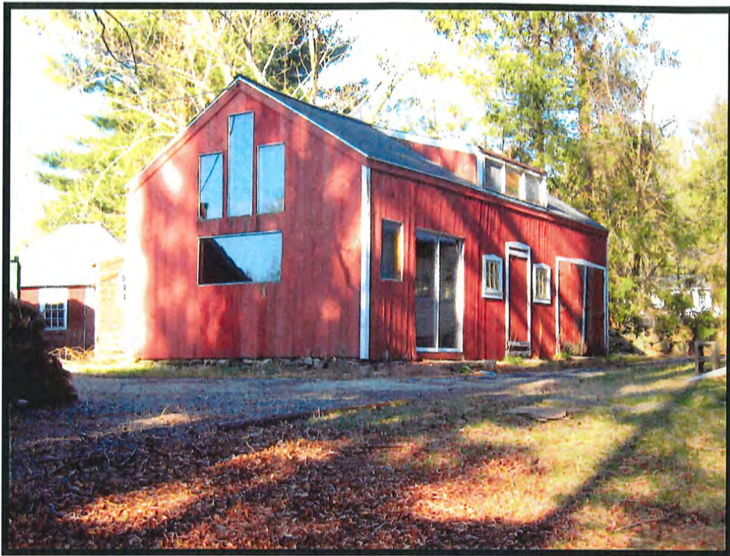
Figure 6. Converted Barn—View to Northeast [B]
