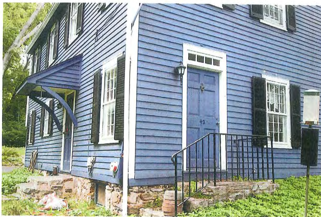
Photo 2. 42 Compo Road North, view east showing side door.
