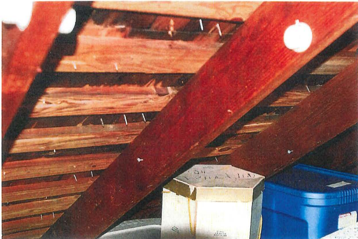
Photo 6. Saltbox roof construction.
