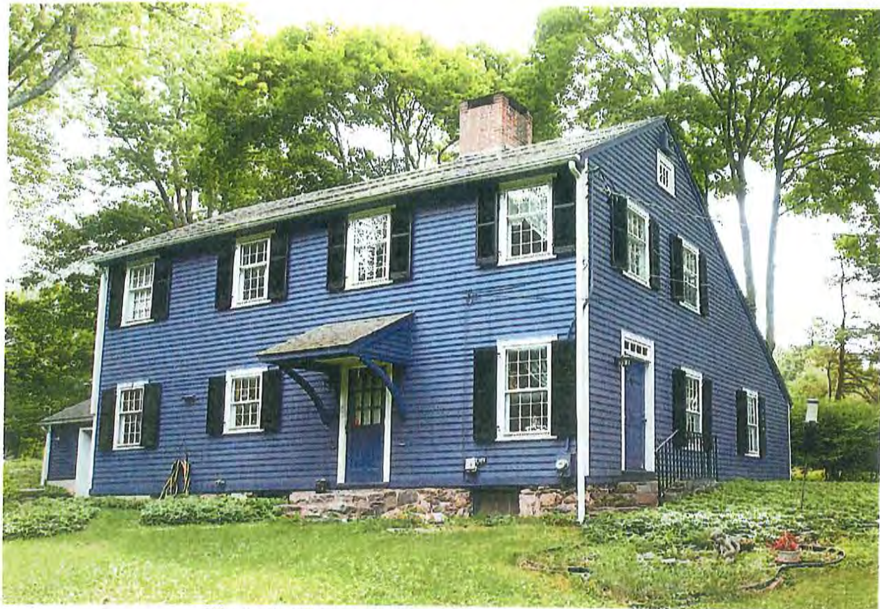
Photo 1. 42 Compo Road North, view southeast.
