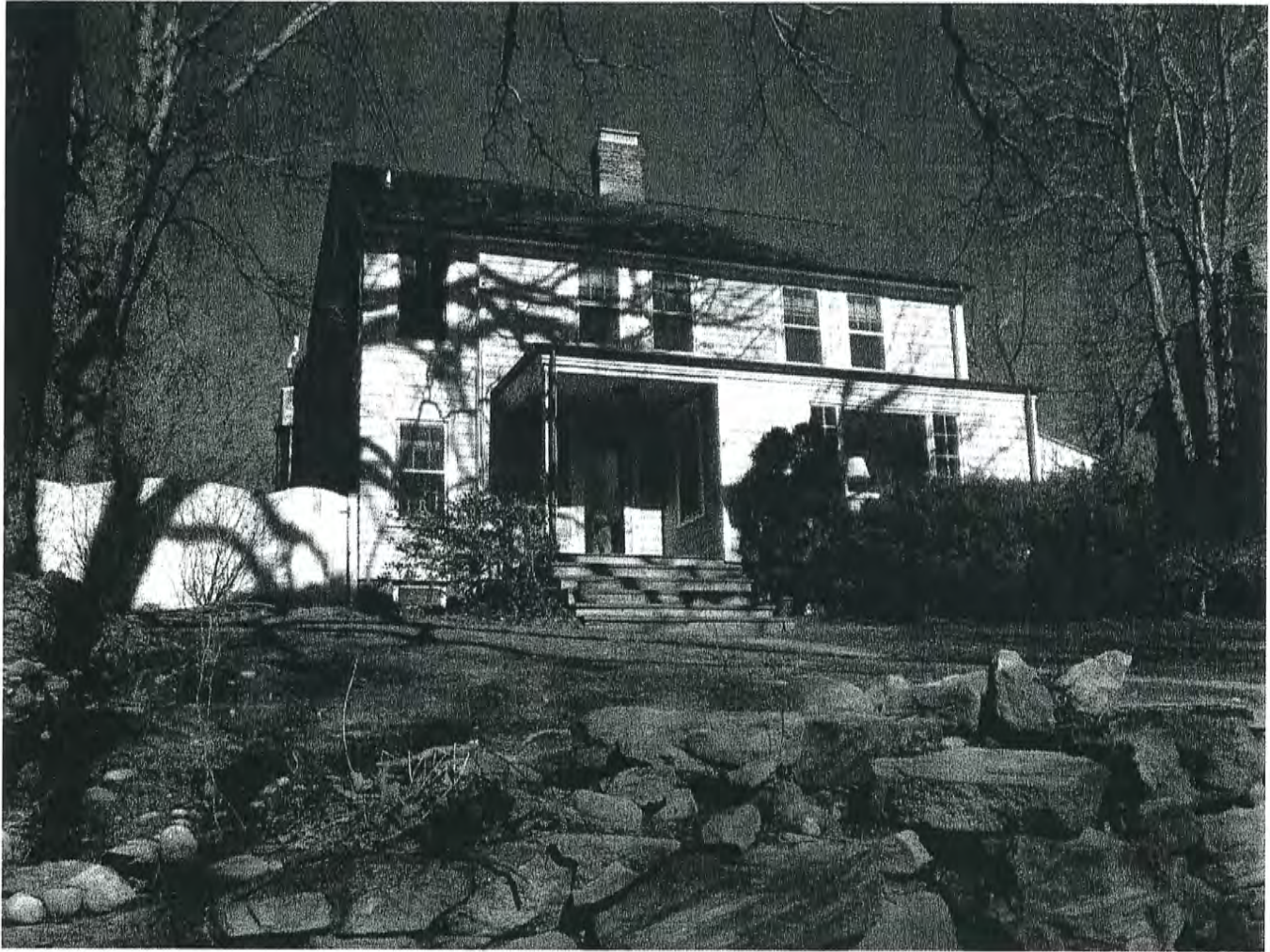
290 Main Street Westport, CT View to East
