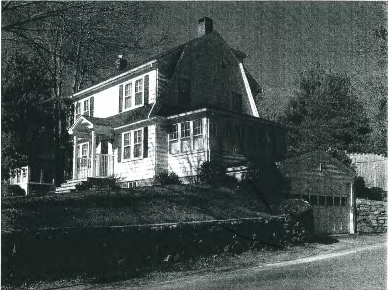
286 Main Street Westport, CT View to East
