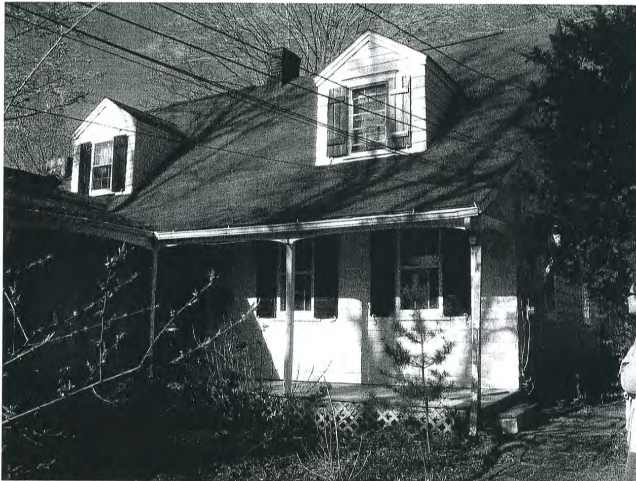
280 Main Street Westport, CT View to East
