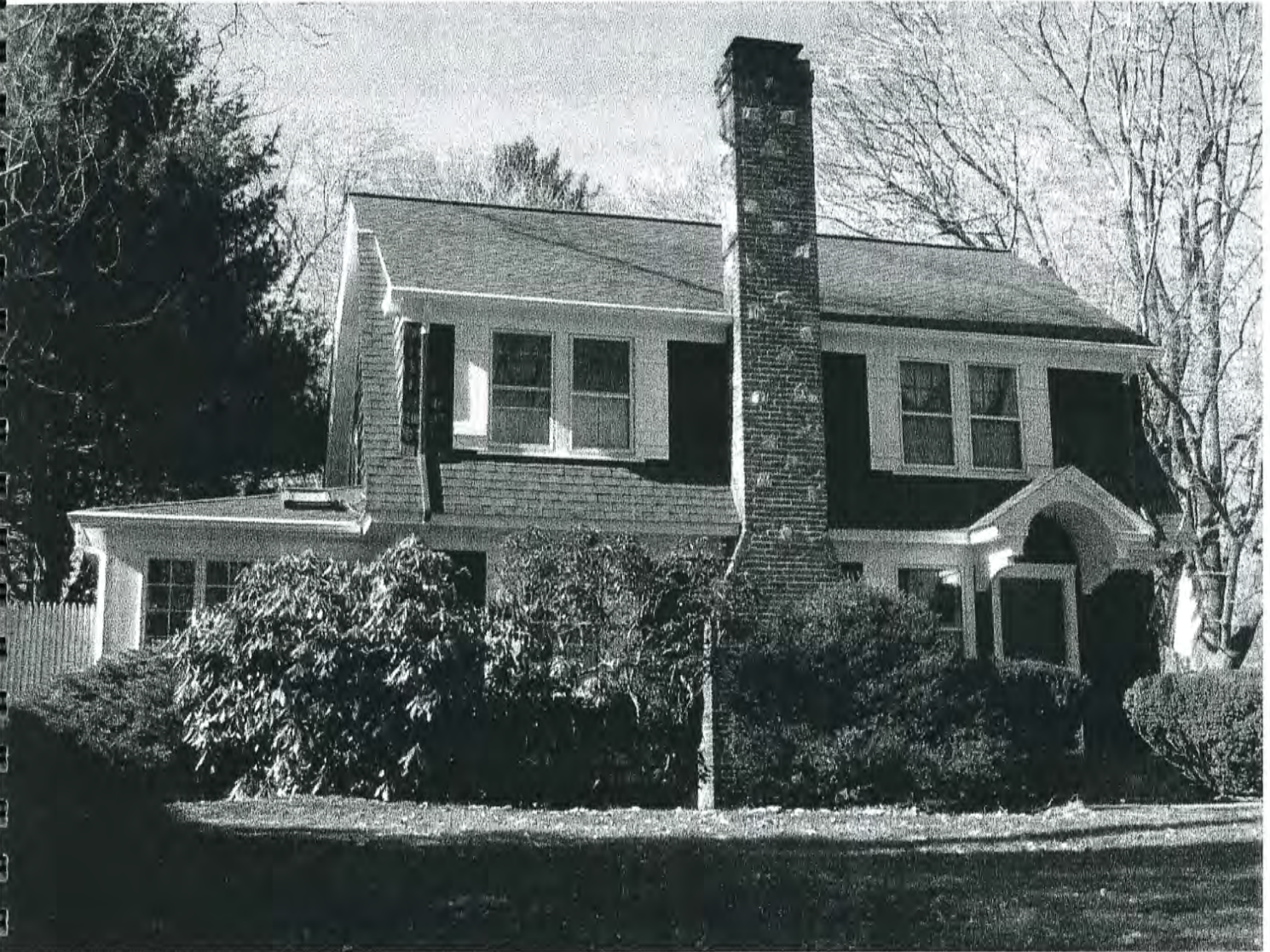
3 Gorham Avenue Westport, CT South Elevation; View to North
