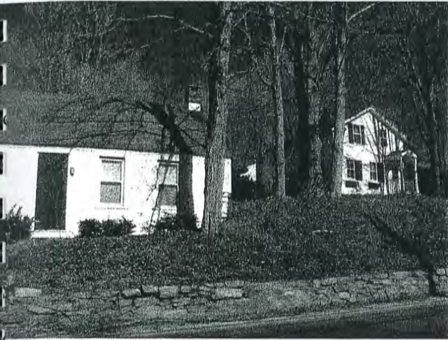
300 Main Street Wesport, CT View to East
