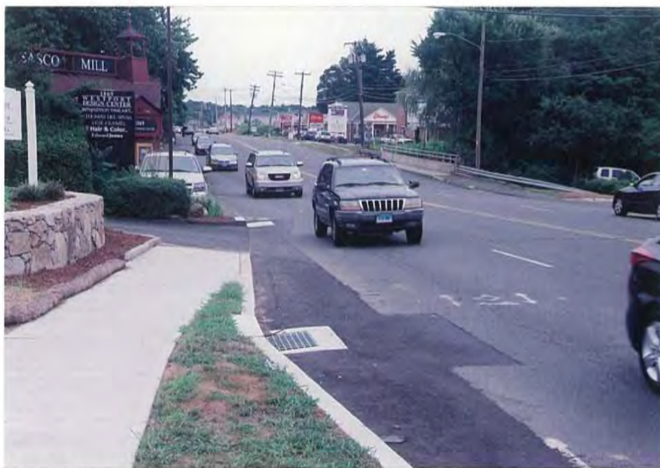
Photo 1-15: Post Road catch basins collect stormwater from the road surface and a system of underground pipes carries the runoff to Sasco Brook.
