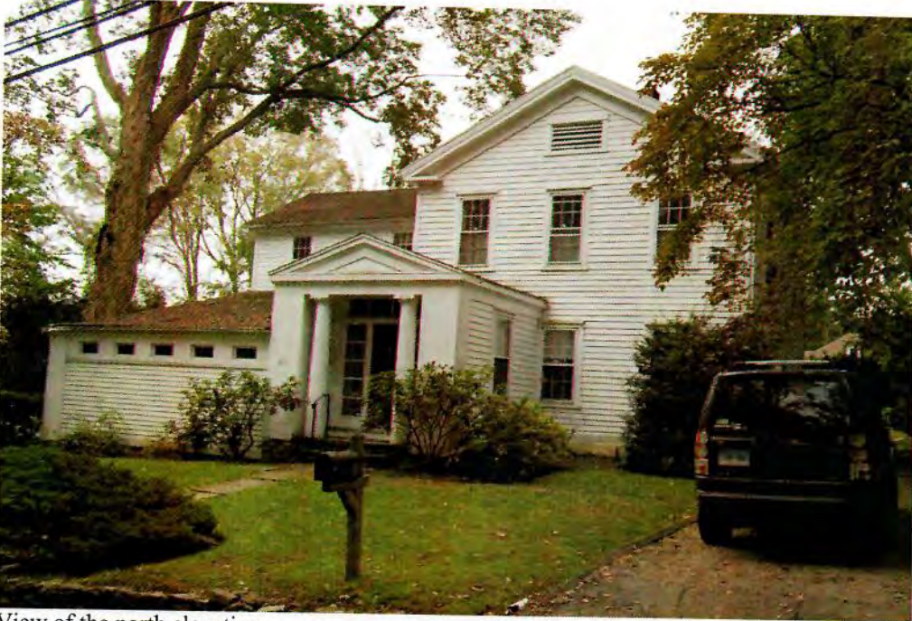
View of the north elevation.
