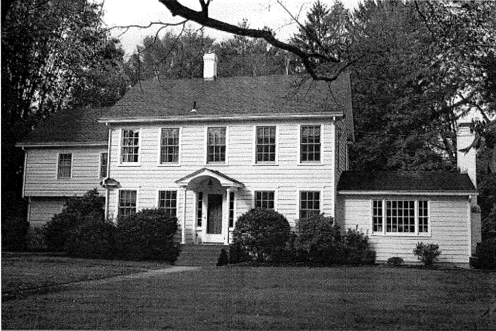
View of the west elevation.
