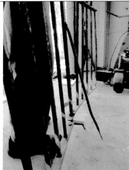
37. Side detail of an original fence post and rail plate joining two rail ends. The rails are bent and broken and existing repairs failing.
