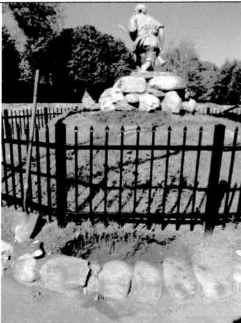
11. Removal of earth that has piled over the outer wall and distribution back to the top of the monument. The stones were solidly set. A lower foundation extended beyond the top footprint.
