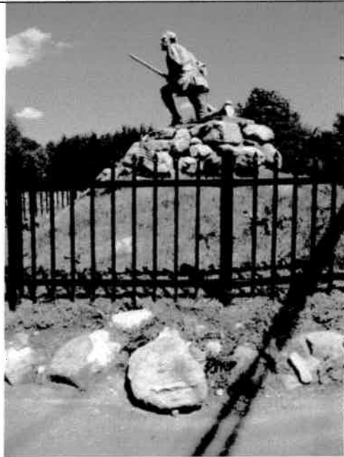
12. View of dislodged perimeter capstones. Most of the stones displaced or damaged occurred at sites of original fence posts.
