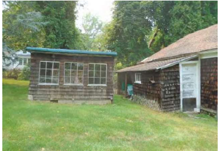
SHED FRONT (EAST)
