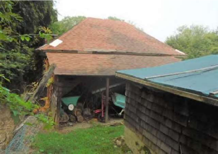
COTTAGE SHED (WEST)
