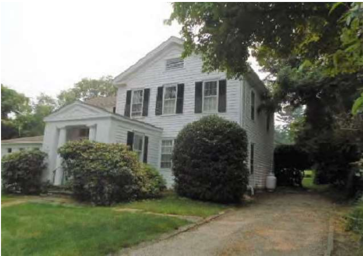
STREET (NORTH) AND SIDE (WEST)
