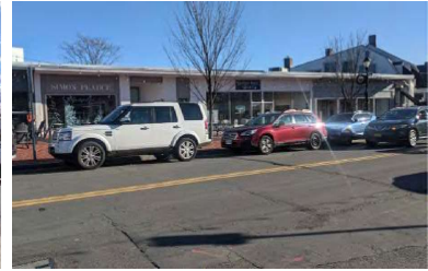
2 NEIGHBORING BUILDINGS - NORTH
