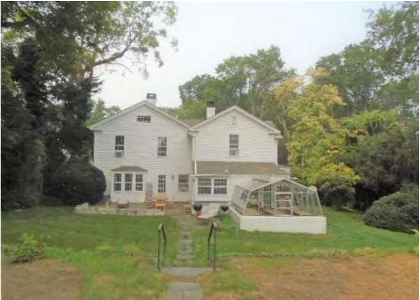
SITE HOUSE (LOOKING NORTH)
