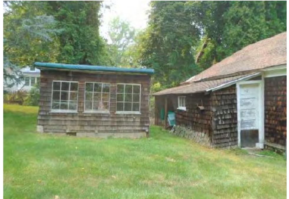
SHED FRONT (EAST)
