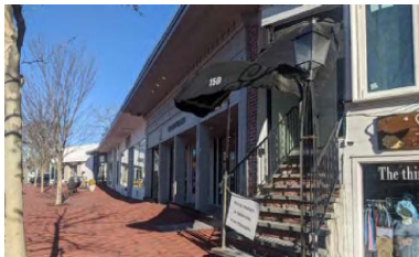
5 NEIGHBORING BUILDINGS - SOUTH
