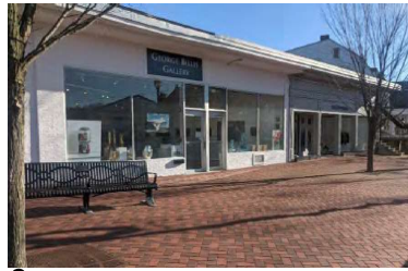
3 NEIGHBORING BUILDINGS - SOUTH
