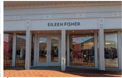
4 NEIGHBORING BUILDINGS - SOUTH
