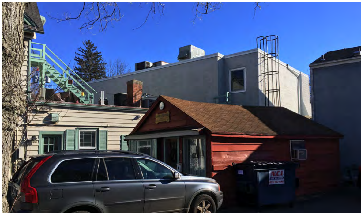
3 PHOTO OF SOUTH FACADE NOT TO SCALE
