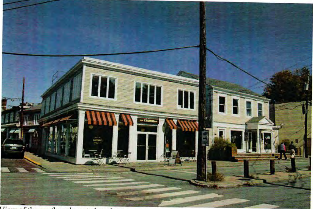
View of the south and west elevations.
