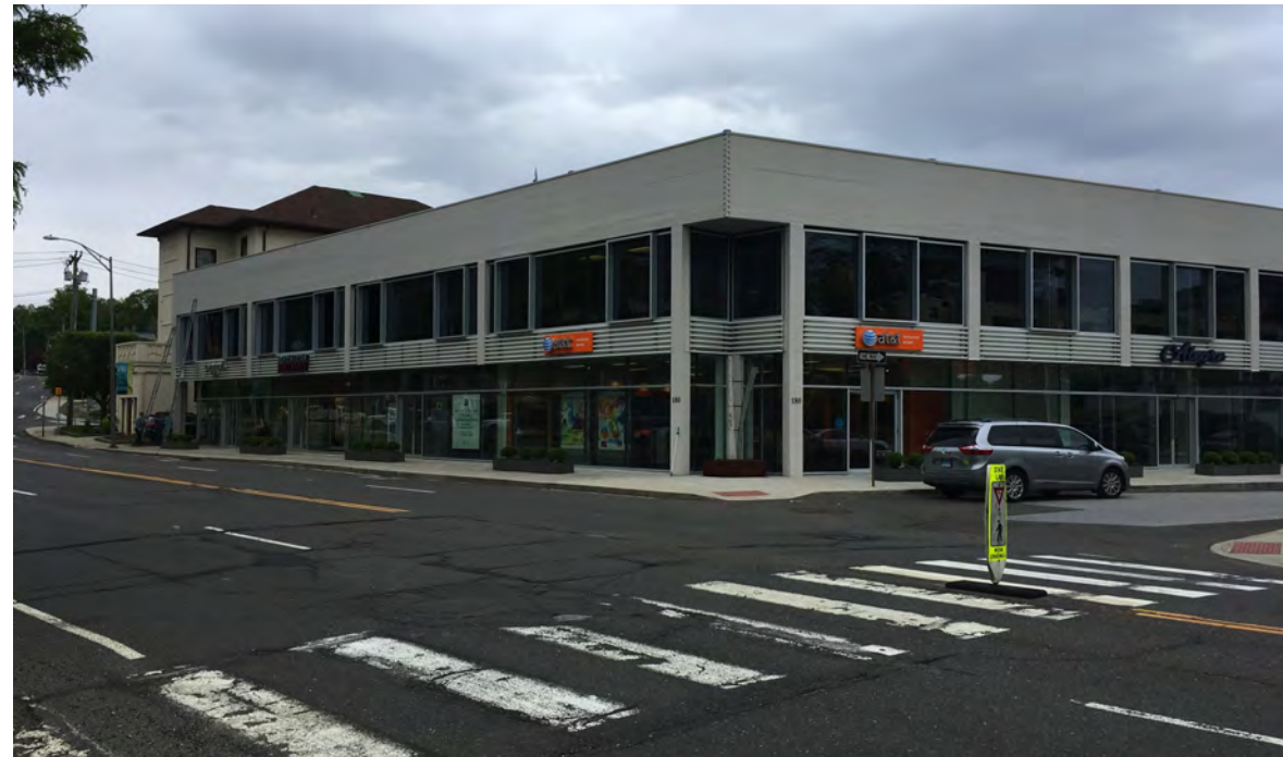
4 PHOTO OF NEIGHBORING BUILDING (POST ROAD) NOT TO SCALE
