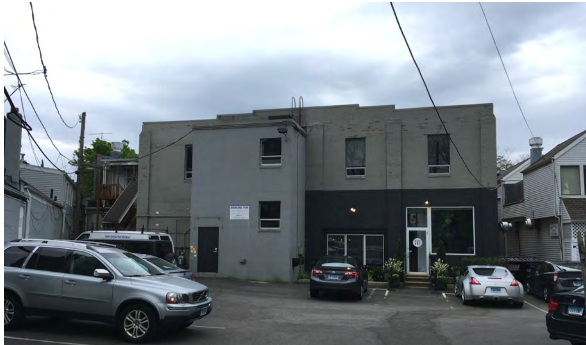
3 PHOTO OF NEIGHBORING BUILDING (BEHIND SITE) NOT TO SCALE
