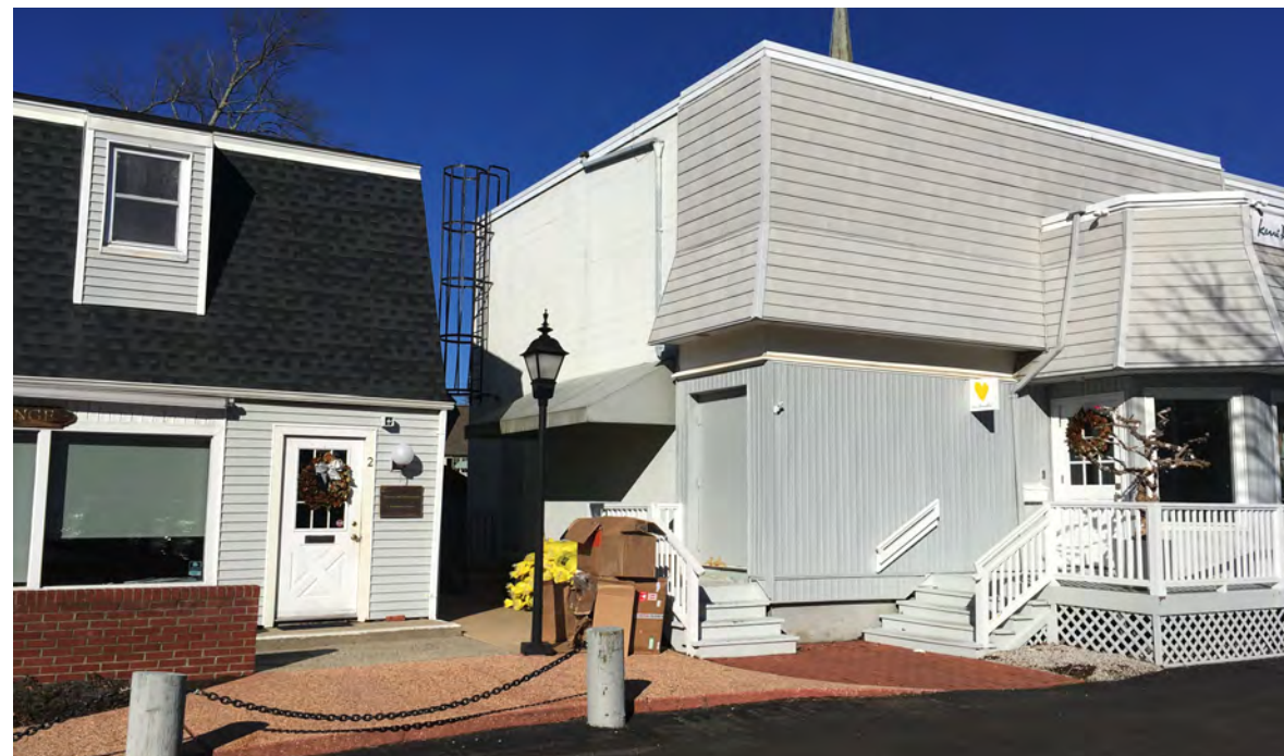
4 PHOTO OF WEST FACADE NOT TO SCALE
