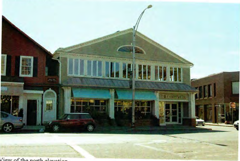
View of the north elevation.
