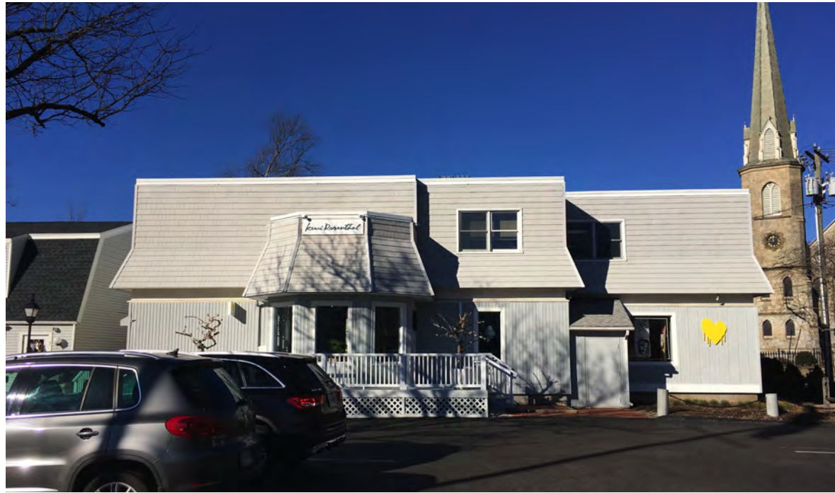
1 PHOTO OF NORTH FACADE NOT TO SCALE
