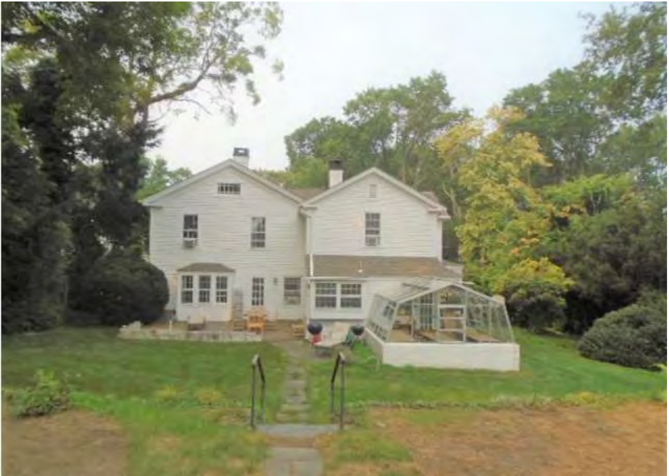
SITE HOUSE (LOOKING NORTH)
