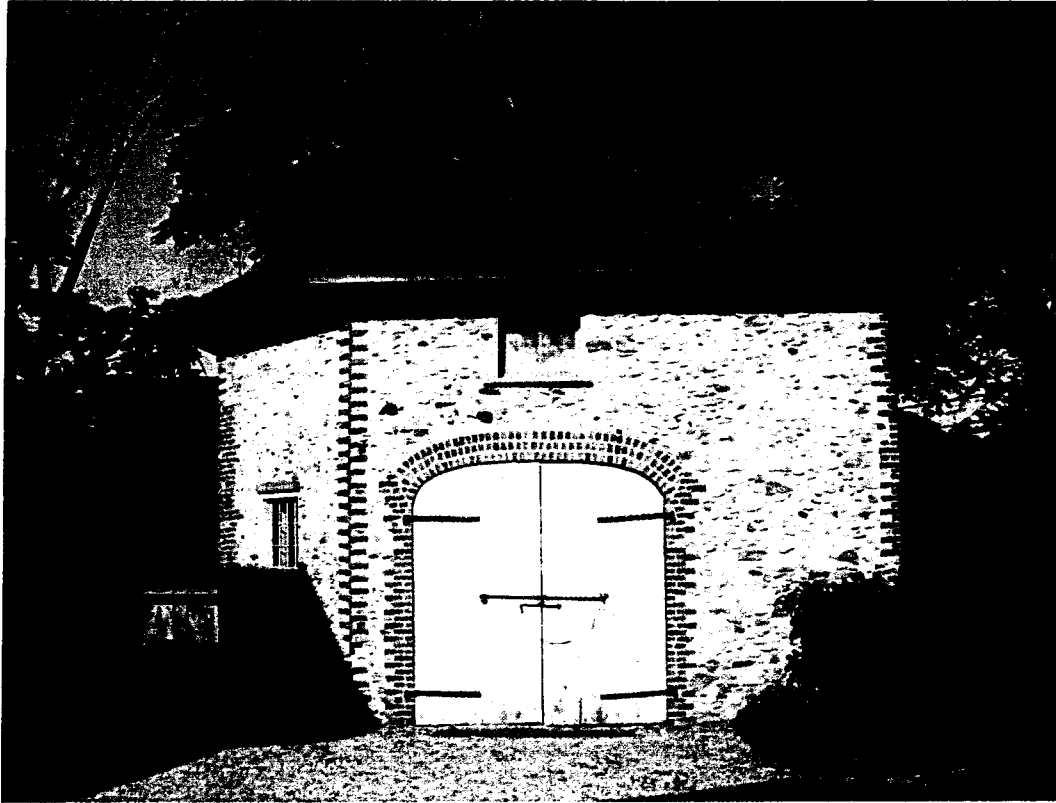
Figure 5: Cobblestone Barn – entrance/east side (2012)
