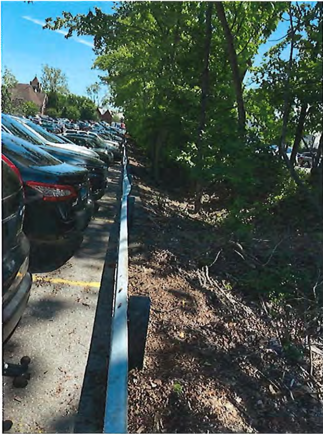
Ditch along West side of lot
