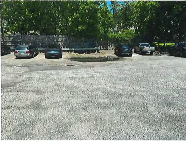
Poor Drainage area rear of lot
