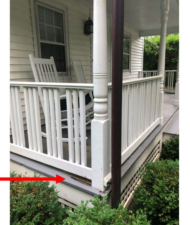
Wood rot/water damage on the front left corner of the porch, likely due to drain spout and exposure to elements. Wood would be replaced and painted to match identically to nondamaged portion of the porch.
