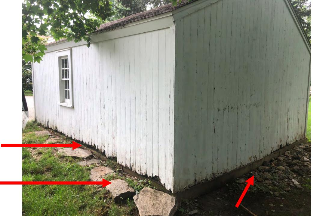
Side elevation of garage to illustrate the 5 ½" new white wood panel that will be added in place of the deteriorating wood.
