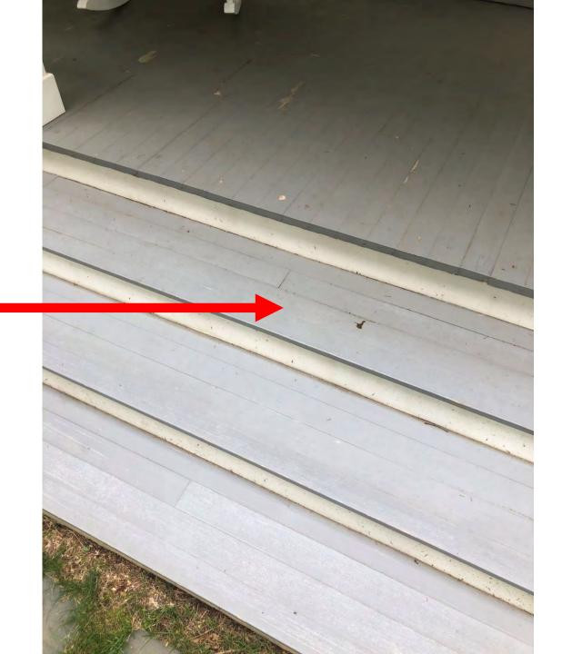
Steps on front porch are sagging at some seams, which are near breaking when someone steps on it 'just so.' The steps need to be reinforced underneath. Visible portion would look identical to what is there currently.
