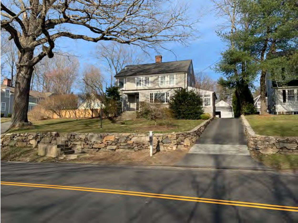
Street frontage with adjacent properties (286 & 296 Main St)
