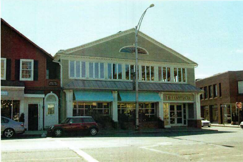
View of the north elevation.
