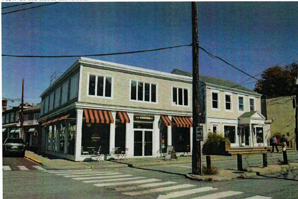
View of the south and west elevations.
