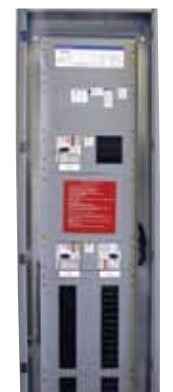
Wall-mount maintenance bypass panel
