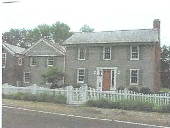
Current house, right side preserved, left side section and garage new.
