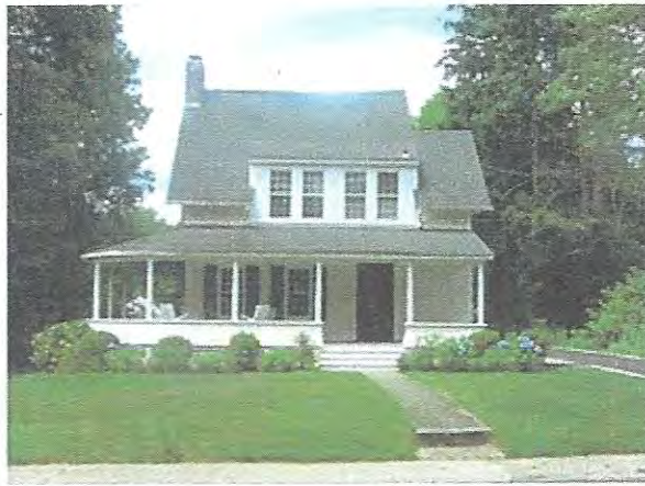
6-30-2019 restored and preserved. Columns required code updating, Bottom shingles hand remade.
