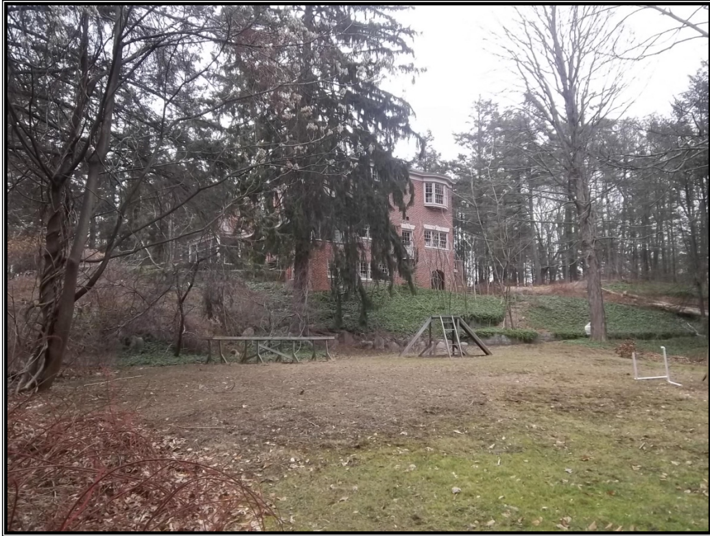
View of existing structure on site
