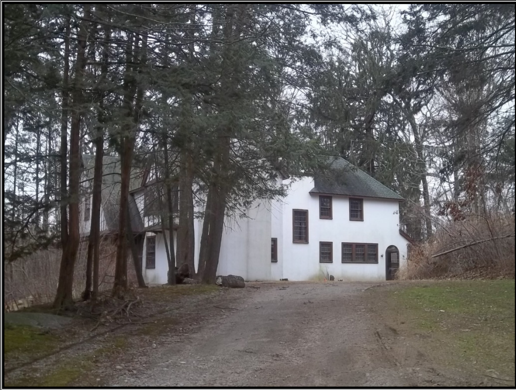
View of existing structure on site
