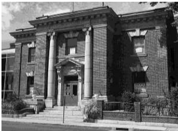
Former Westport Library, 1908
