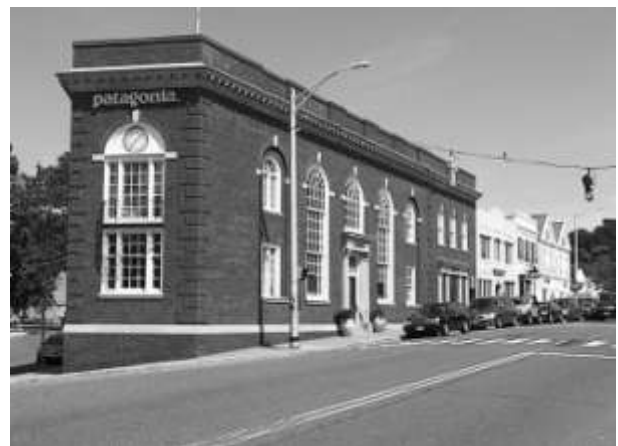
Former Westport Bank & Trust, by Charles E. Cutler; Architect, 1924
