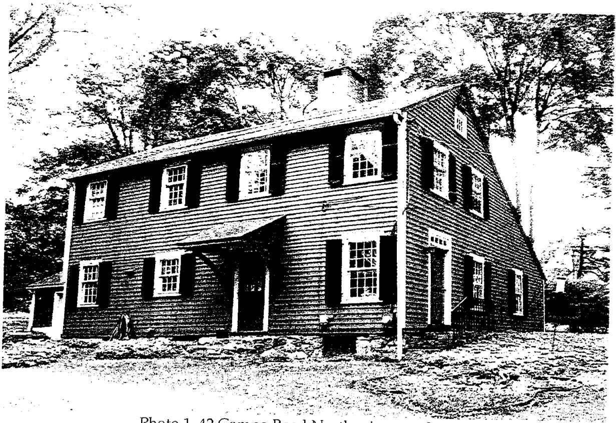
Photo 1. 42 Compo Road North, view southeast.
