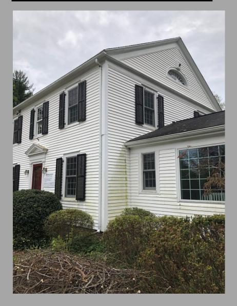
Original wood clapboard siding has been replaced by vinyl siding, vinyl corner boards, and trim details. Asphalt shingle roof. Plastic and vinyl eaves and soffits.
