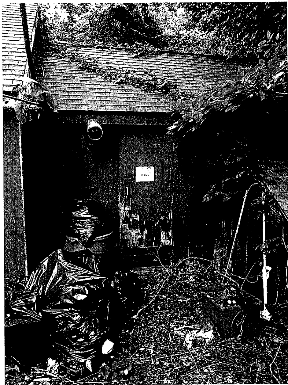
Rotted siding, bottom of door rotted out, animal entrance
