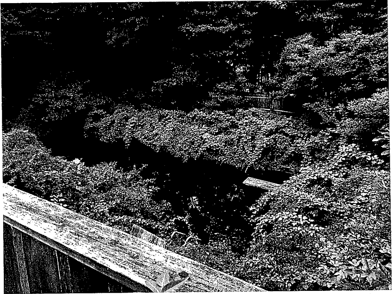
Pool with overgrown vegetation; NO maintenance done for at least a decade
