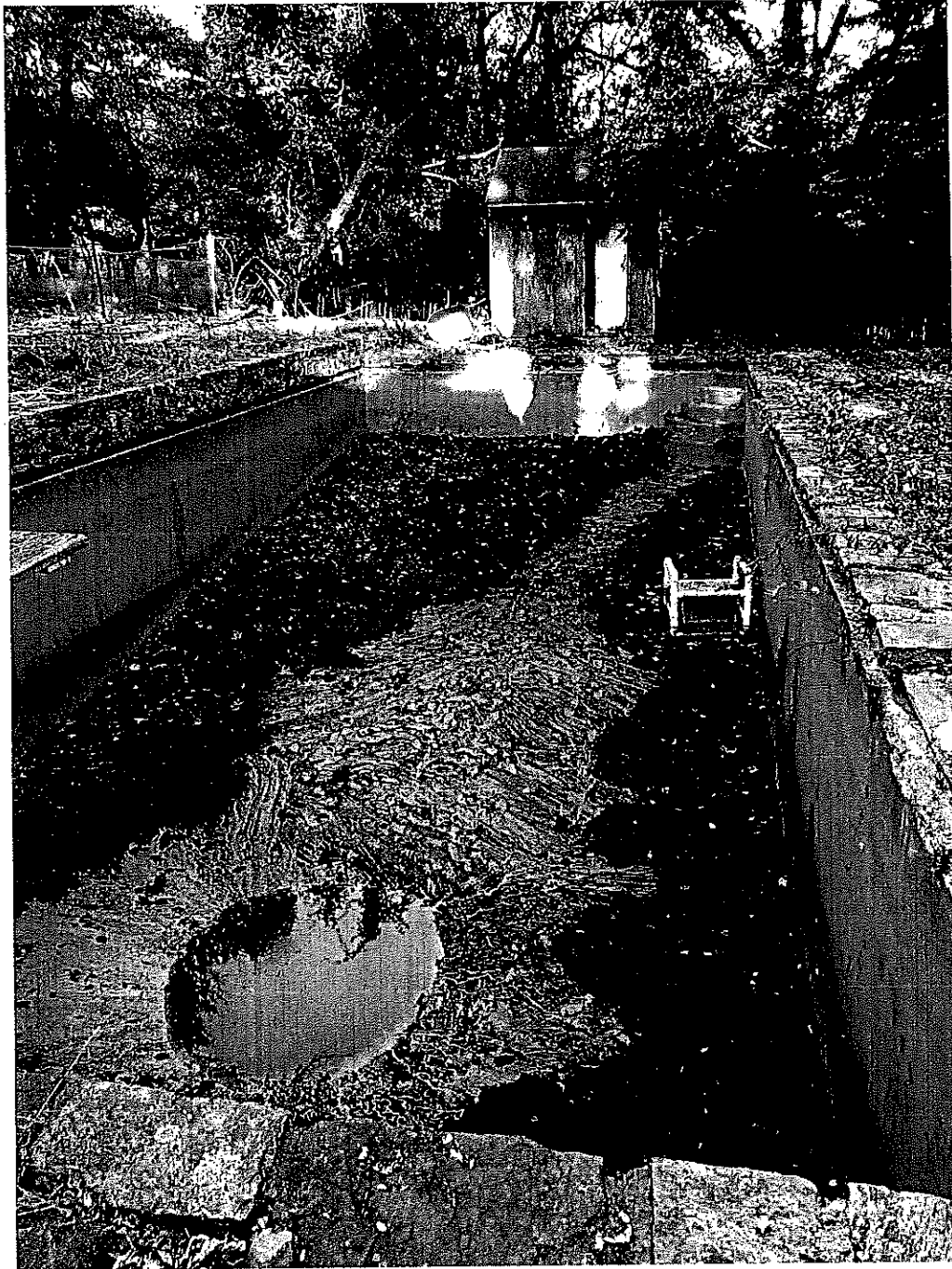
This is what the pool looked like after draining. This is NOT a $50,000 pool. No tiling, no coping, no decking, just rough stone around the edge, no heater, no functioning filter.
