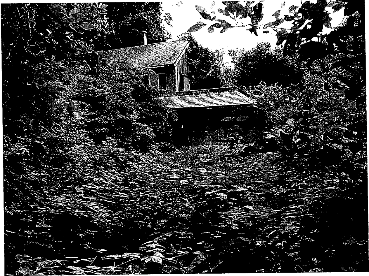
Vines growing INTO the house, siding missing just below 'terrace'
