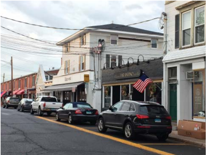
Existing parking conditions along Railroad Place.
