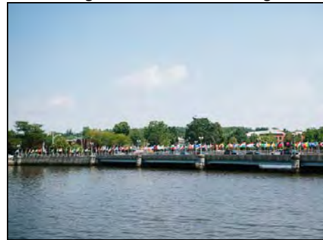
Rising Water At Post Road Bridge
