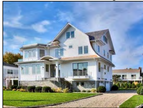
House Elevated To Flood Height
