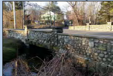
Greens Farm Road Bridge
