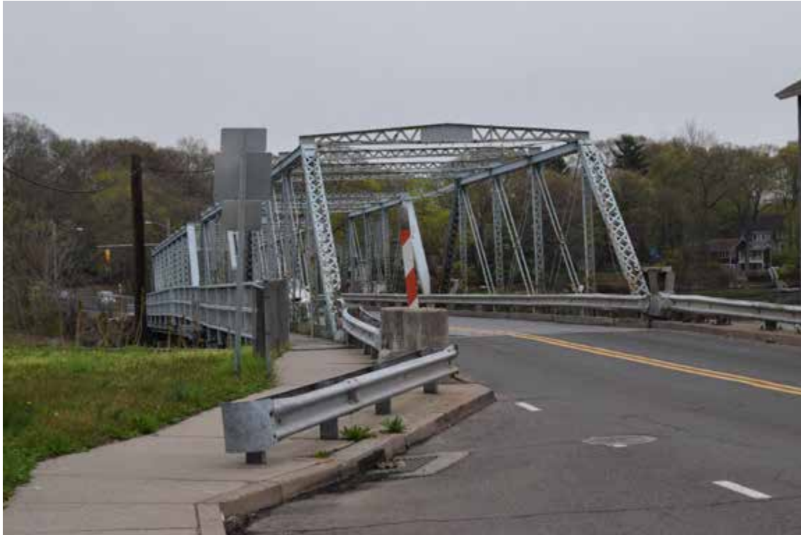
Photo 27. Saugatuck River Swing Bridge, looking east.
