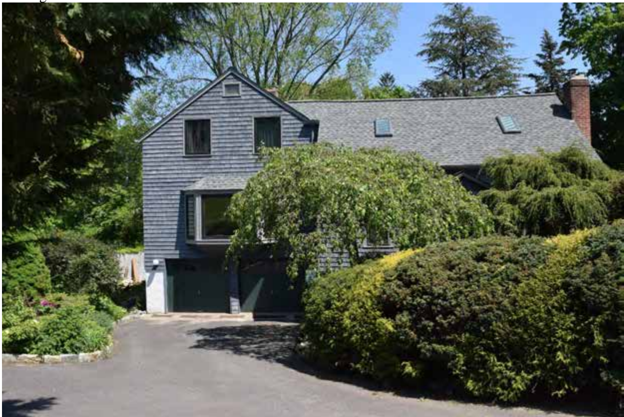
Photo 10. Lyons House, 27 Bridge Street, looking east.
