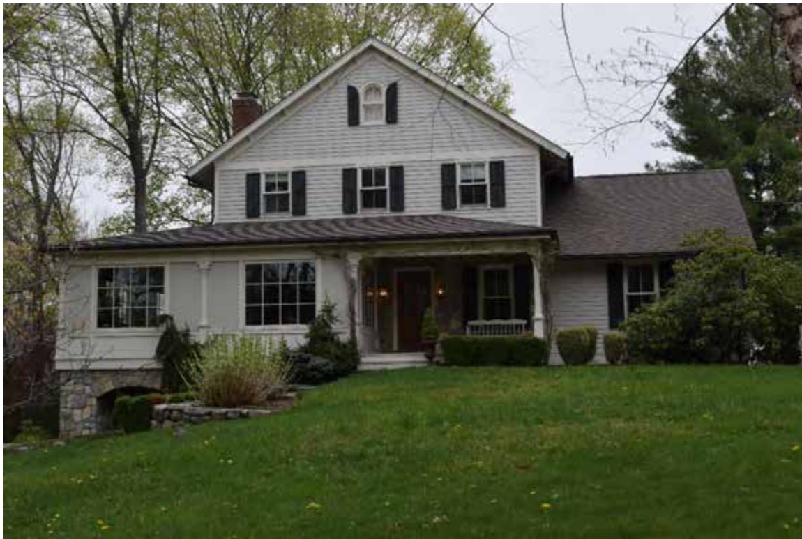
Photo 16. 17 Bridge Street, looking north.
