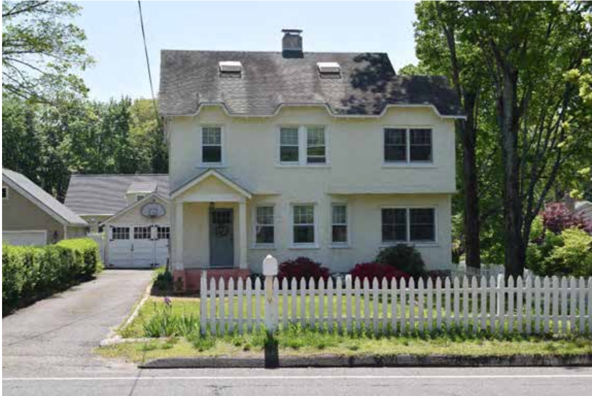
Photo 7. Joseph Postorino House, 32 Bridge Street, looking south.
