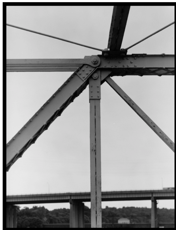
Figure 15. Eye Bar Detail (HABS, 1968)
