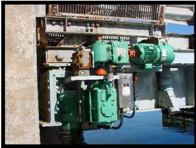
Figure 12. Detail of Special Screw Jack Assembly
