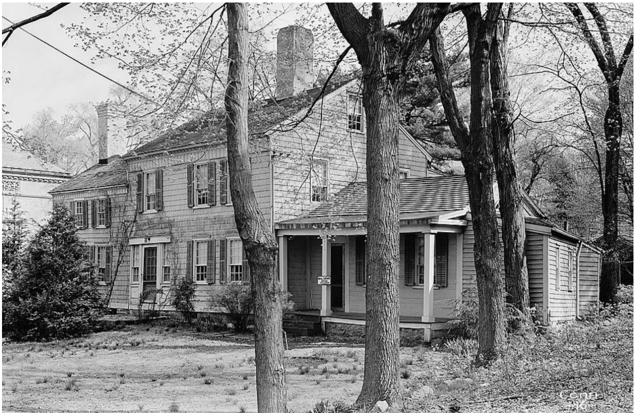
The Dunn House along Myrtle Ave. was constructed sometime in the early 1800s. (Source: Library of Congress)
