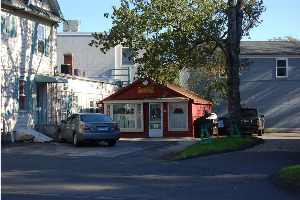
View of the converted garage.
