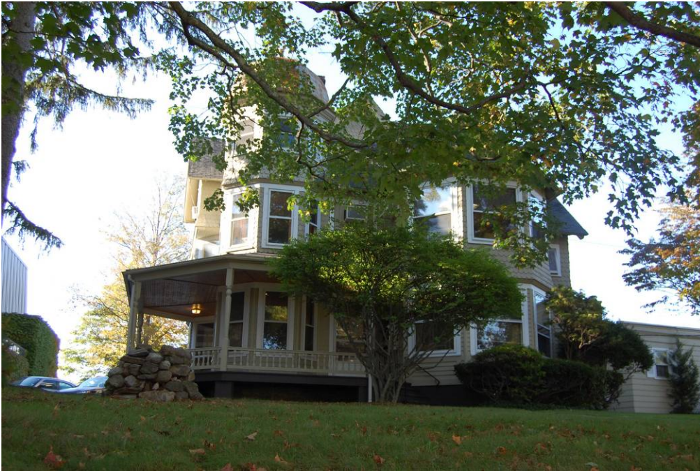
View of the southeast and southwest elevations.
