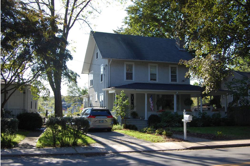
View of the east and south elevations.
