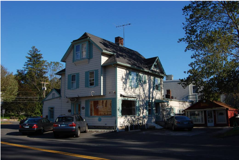
View of the north and west elevations.
