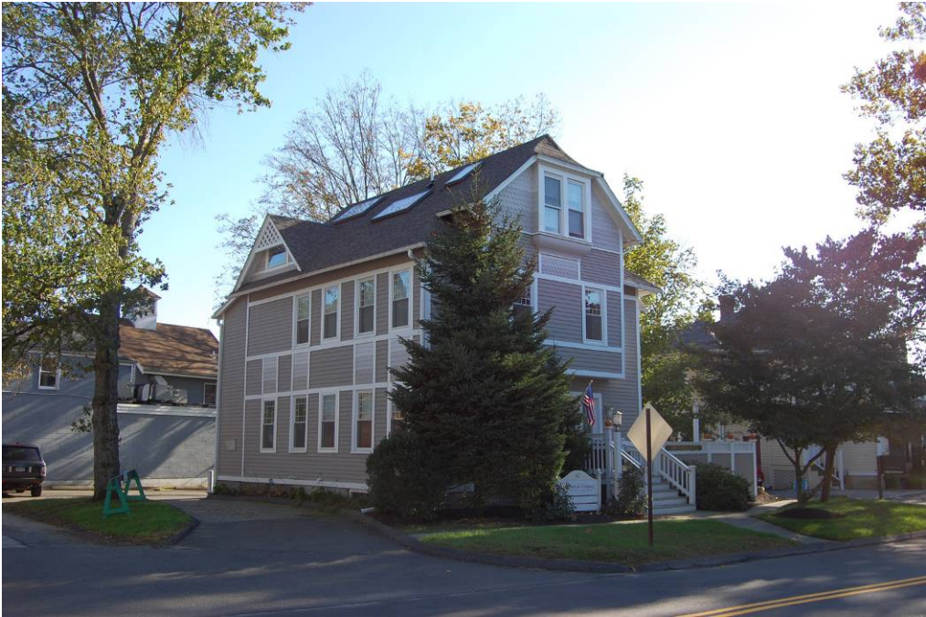
View of the northwest and northeast elevations.
