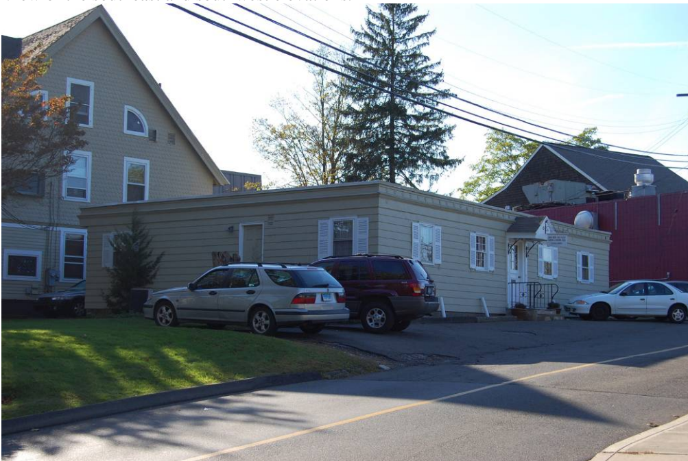
View of the northeast elevation and modern office building.
