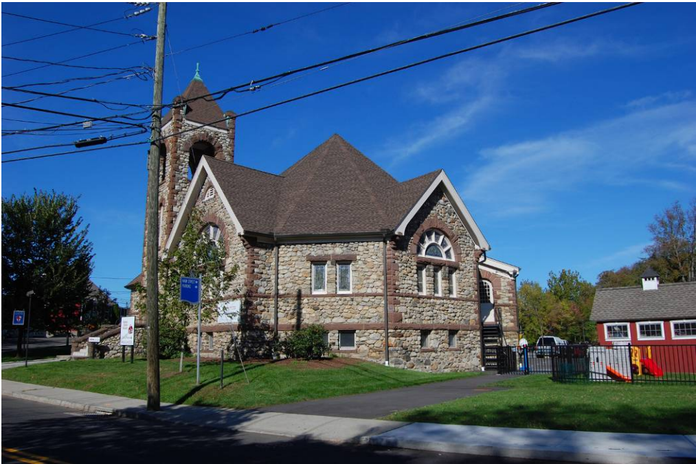
View of the east elevation.
