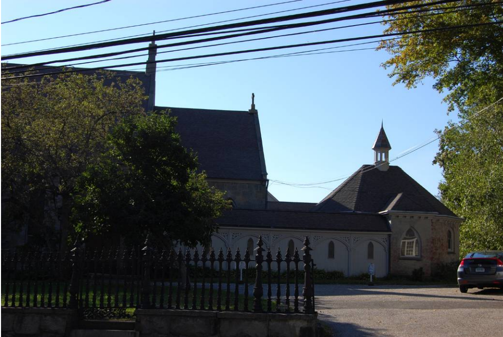
View of the east elevation.
