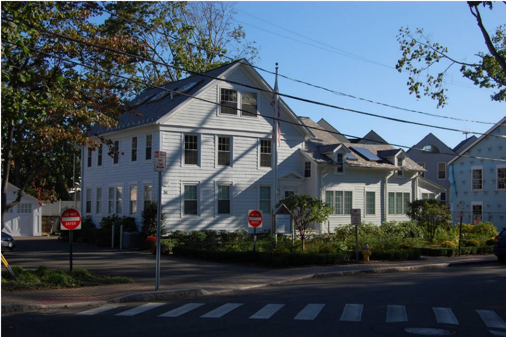
View of the northwest and northeast elevations.
