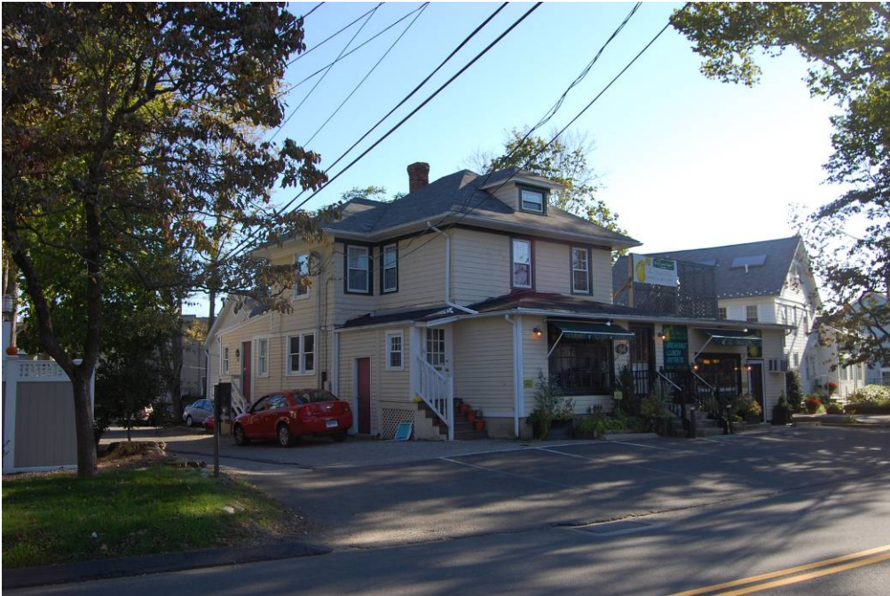
View of the northwest and northeast elevations.
