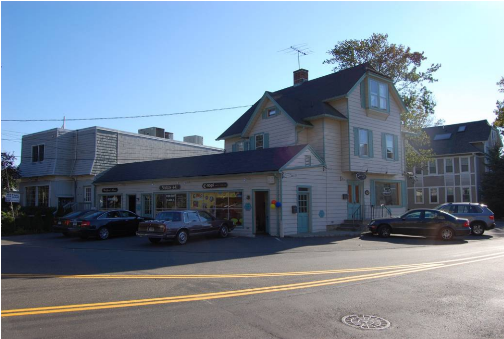
View of the north and east elevations.
