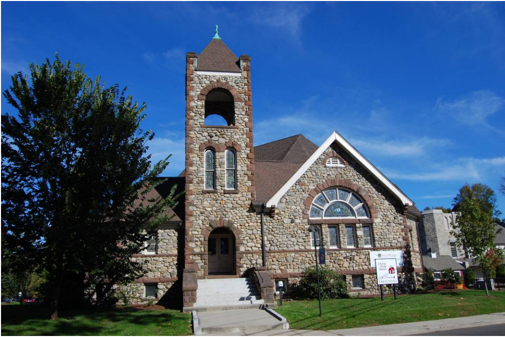
View of the south elevation.
