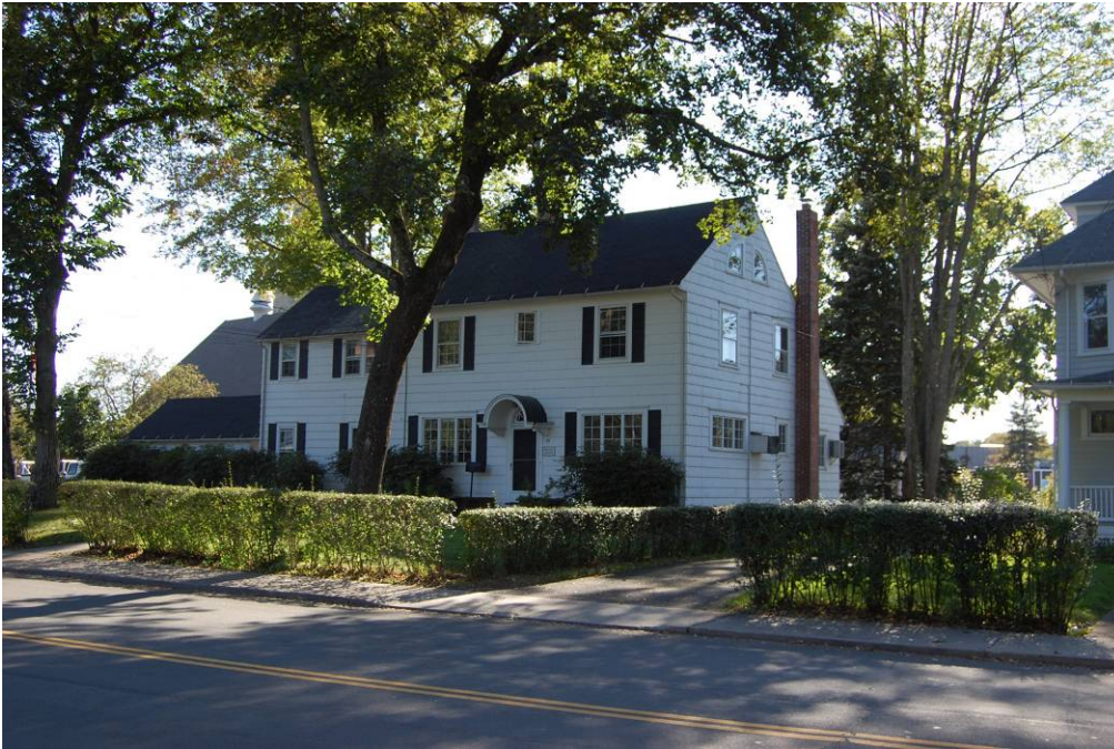
View of the northeast and northwest elevations.
